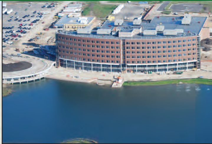
Sherman Hospital Geothermal Lake, Elgin, IL
