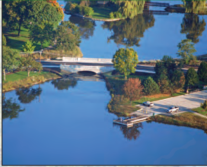
Lake Street Bridge, Libertyville, IL
